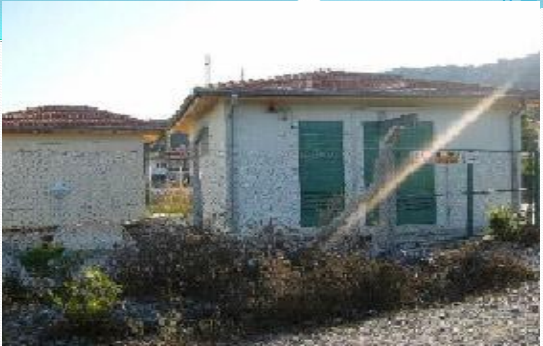
Picture 4: Dalyan Fresh Water Depository
