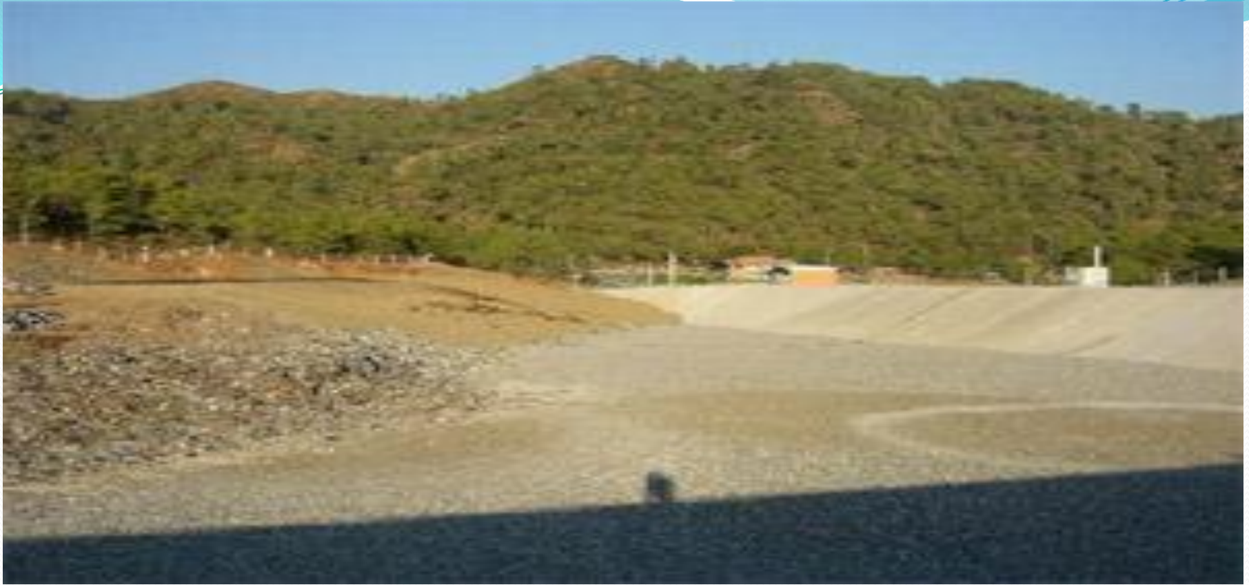
Picture 5:Ortaca Garbage Storage Plant
